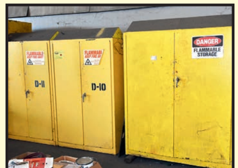
FLAMMABLE MATERIALS STORAGE CABINETS
