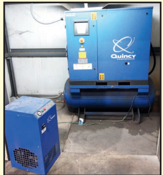
QUINCY 20 HP ROTARY SCREW TYPE AIR COMPRESSOR AND DRYER
