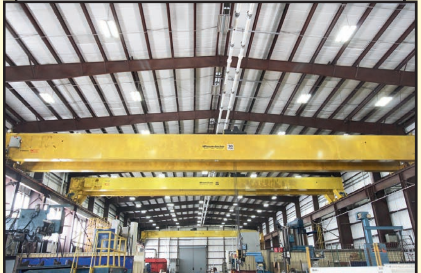
PROSERV 30 T. X 100' SPAN OVERHEAD BRIDGE CRANE
