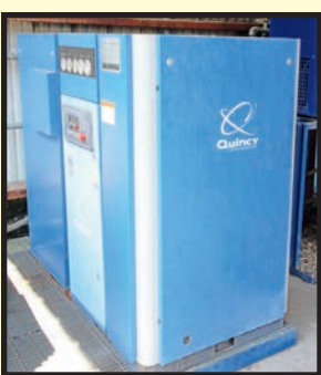
QUINCY ROTARY SCREW AIR COMPRESSOR
