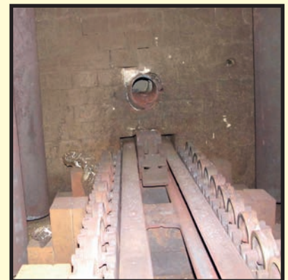
INTERNAL VIEW OF SAUDER INTERNAL QUENCH HEAT TREAT LINE
