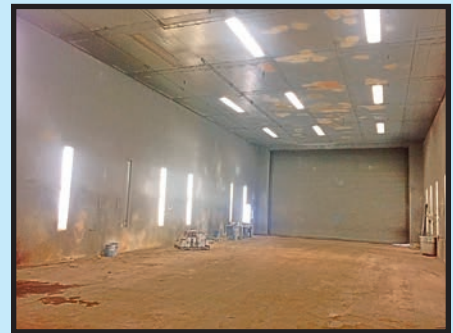
(1) BLAST AND (1) LARGE PAINT BOOTH
