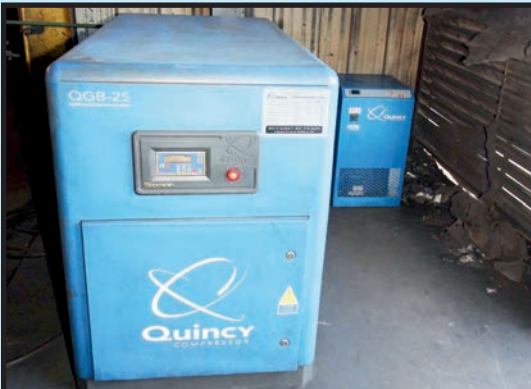
QUINCY MDL. QB25 ROTARY SCREW AIR COMPRESSOR
